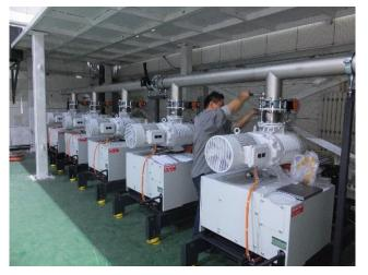
**Cold box and compressor (deliver next week)** refrigeration: 1000 W @ 4.5K, liquefaction: 284 L / h Installed 2K pumps (total) 8000 m<sup>3</sup>/h @ 3100 Pa
