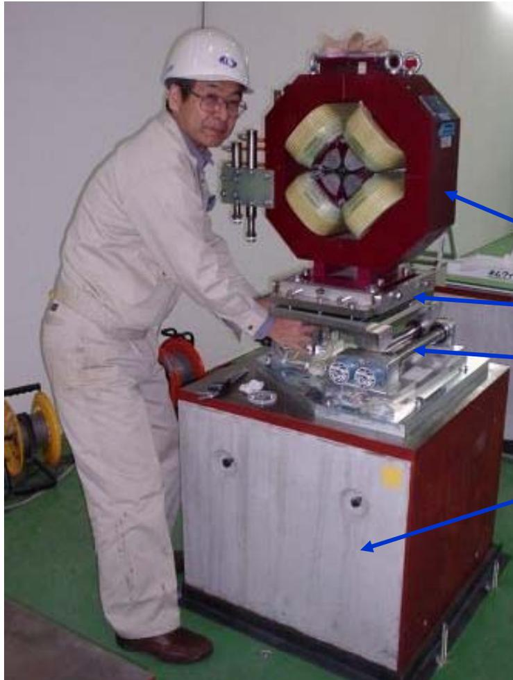
Sugahara-san and small crew is installing the concrete base blocks in the ATF2 beamline.
