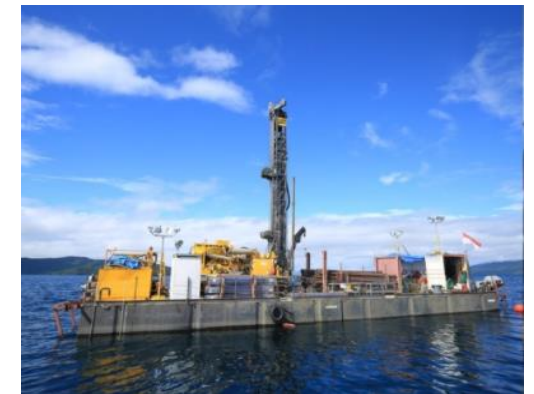
Drilling work on the lake
