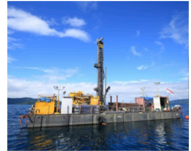
Drilling works on the Lake Geneva
