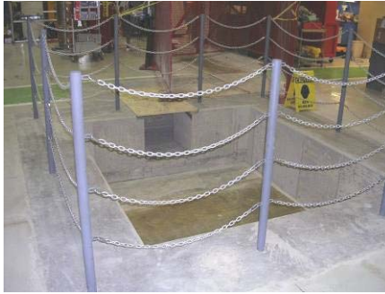
Figure 2: VTS civil construction completed in August 2006
