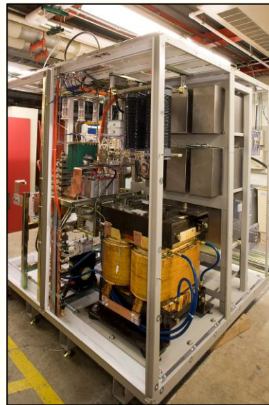
Views of crowbar switch, chokes, and capacitor bank.
