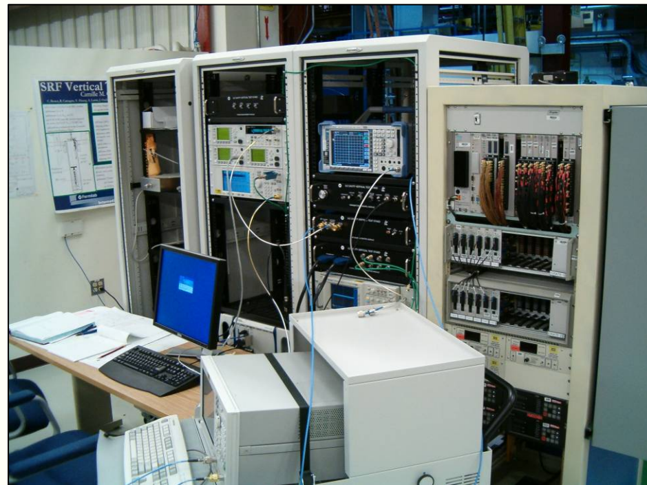
Vertical Test Control Console
