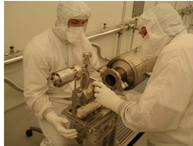
Installation of burst disc/pump-out flange
