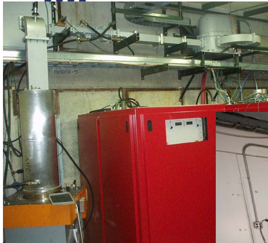
300 kW RF klystron system
