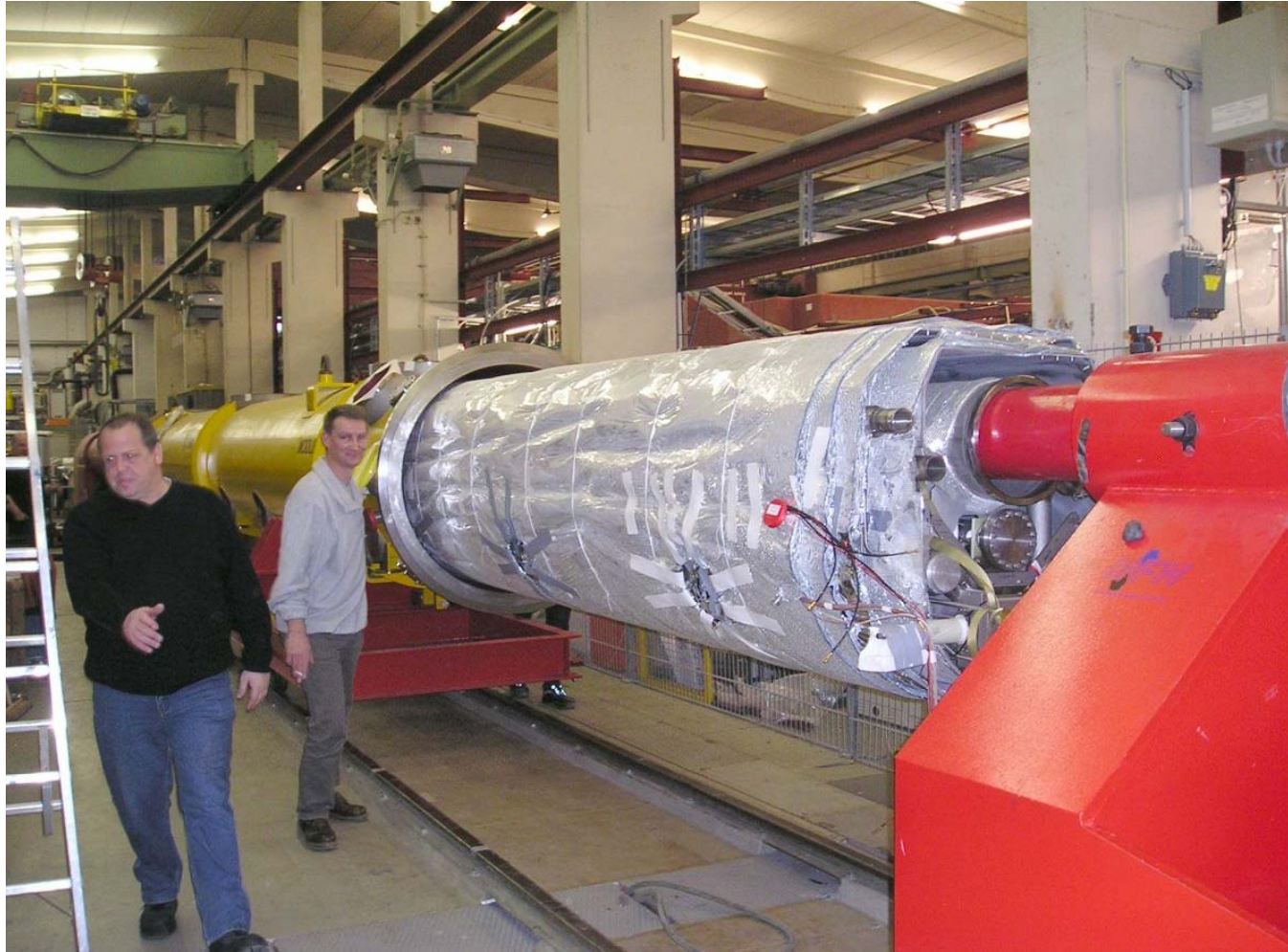
Sliding the Vacuum Vessel
