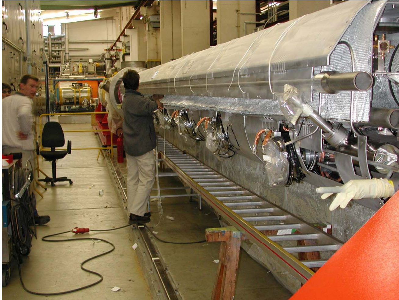
Close internal shield MLI
