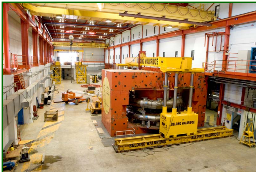
NML During Removal of Chicago Cyclotron Magnet (CCM) (September, 2006)
