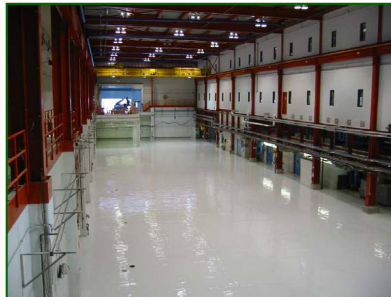
NML Facility after CCM Removal and Floor Painting (February, 2007)
