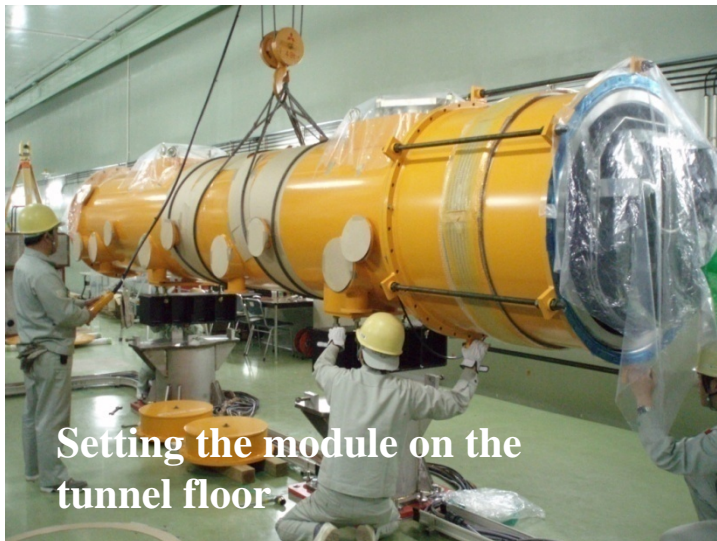
Cold mass hung under the assembly tool
