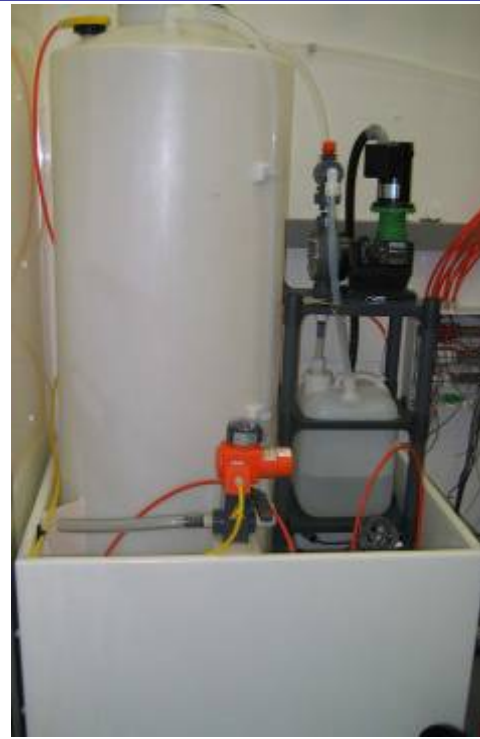
Dilute Waste Neutralization System
