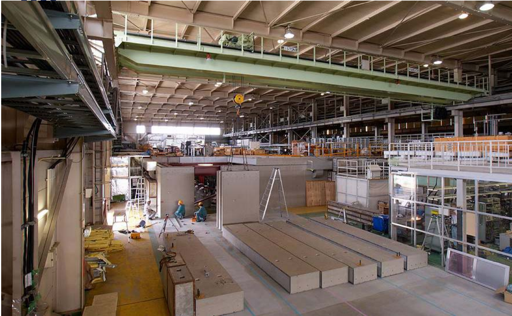
Photos from ATF2 construction, N.Toge
