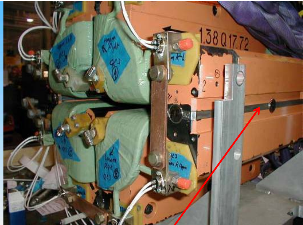
Shims added at split plane
