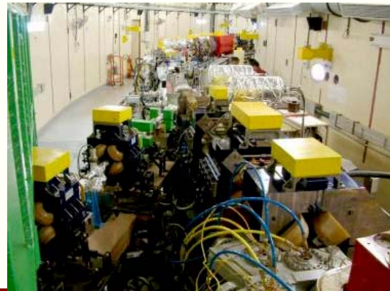
Transport Line-3 Joining on to Indus-2
