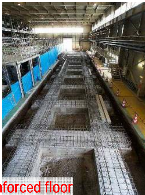
Construction of shielding
