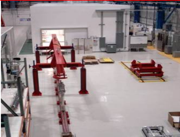
CAF-MP9 Clean Room
