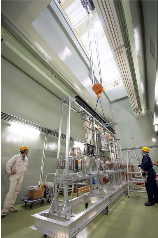
WG unit installation.
