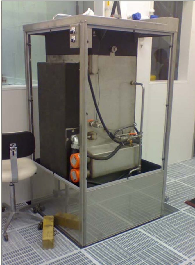
Installation of ultrasonic cleaning system in progress
