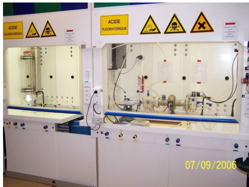
1-cell horizontal EP set-up in operation
