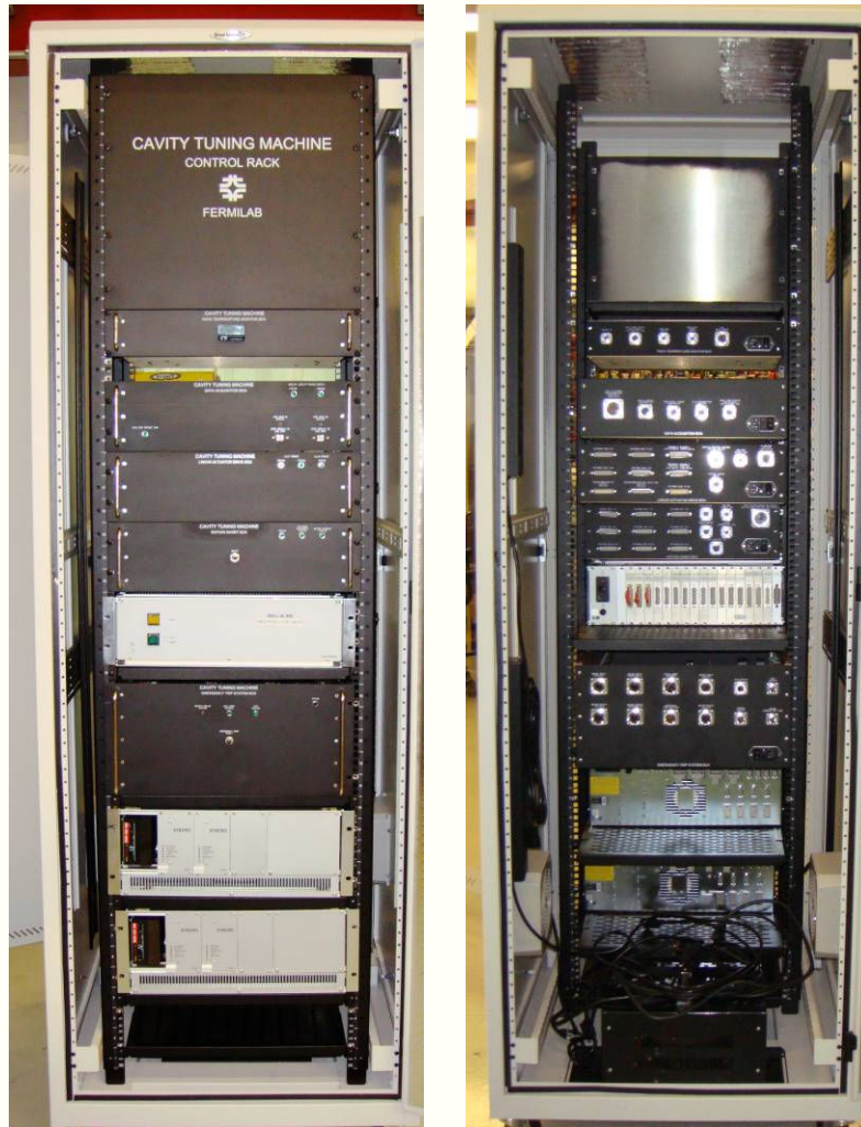
First production control rack fabrication in progress
