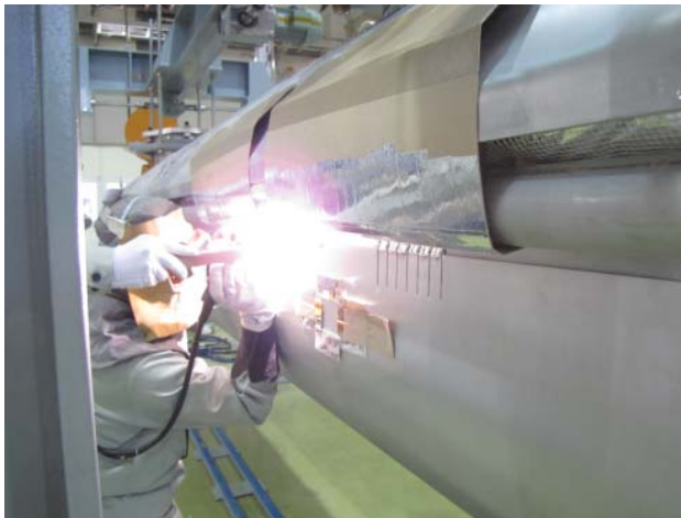
Welding of 5K shield. After welding, all bolts were dismantled.
