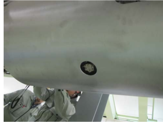
Making holes for FNAL cool-down pipe connection
