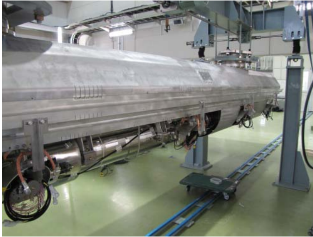
Assembling 5K shield
