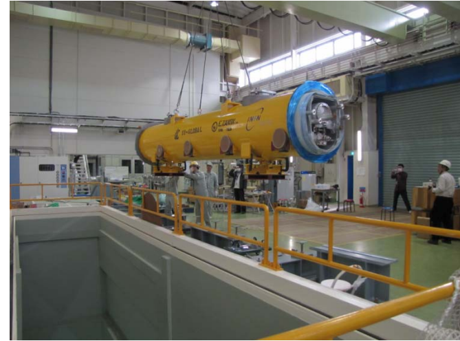
Moving the Module-C into the STF tunnel
