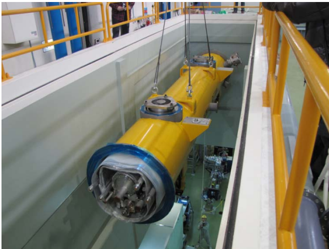
Moving the Module-C into the STF tunnel
