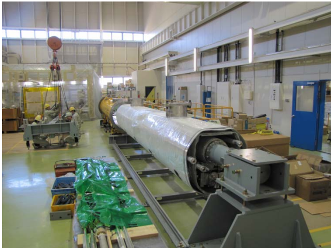
Setting the cold mass on the equipment
