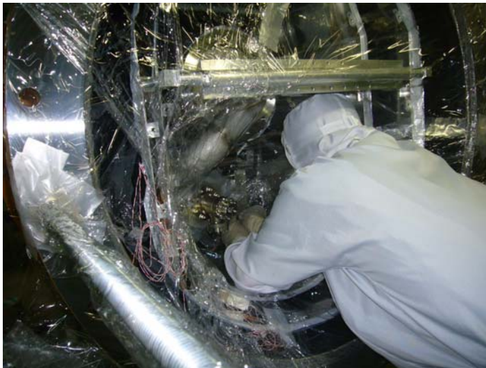
Connection of Beam Tubes
