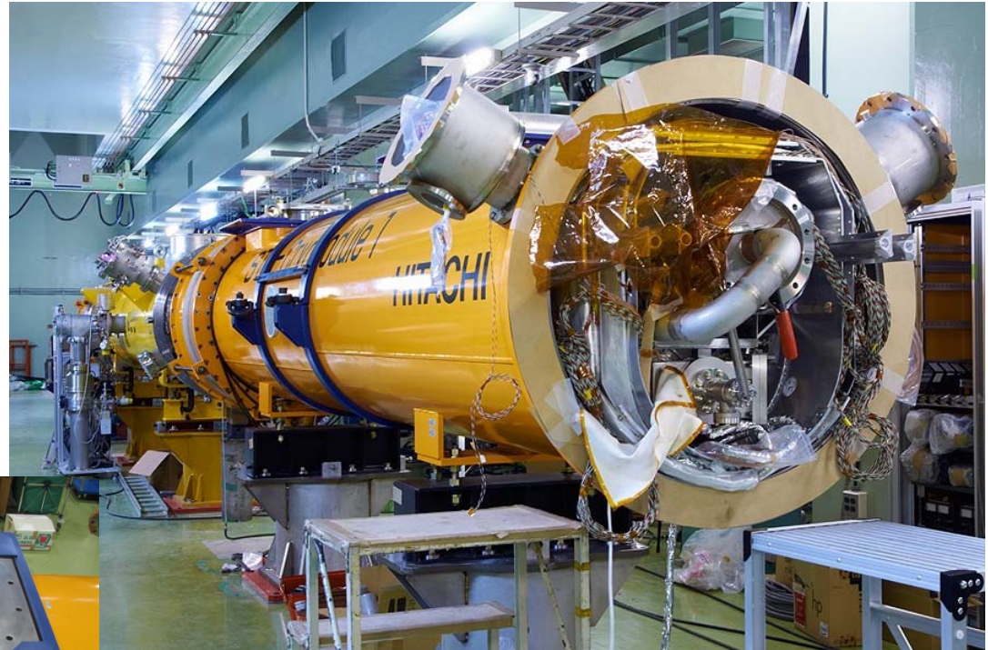
Moving the Module-A into the STF tunnel
