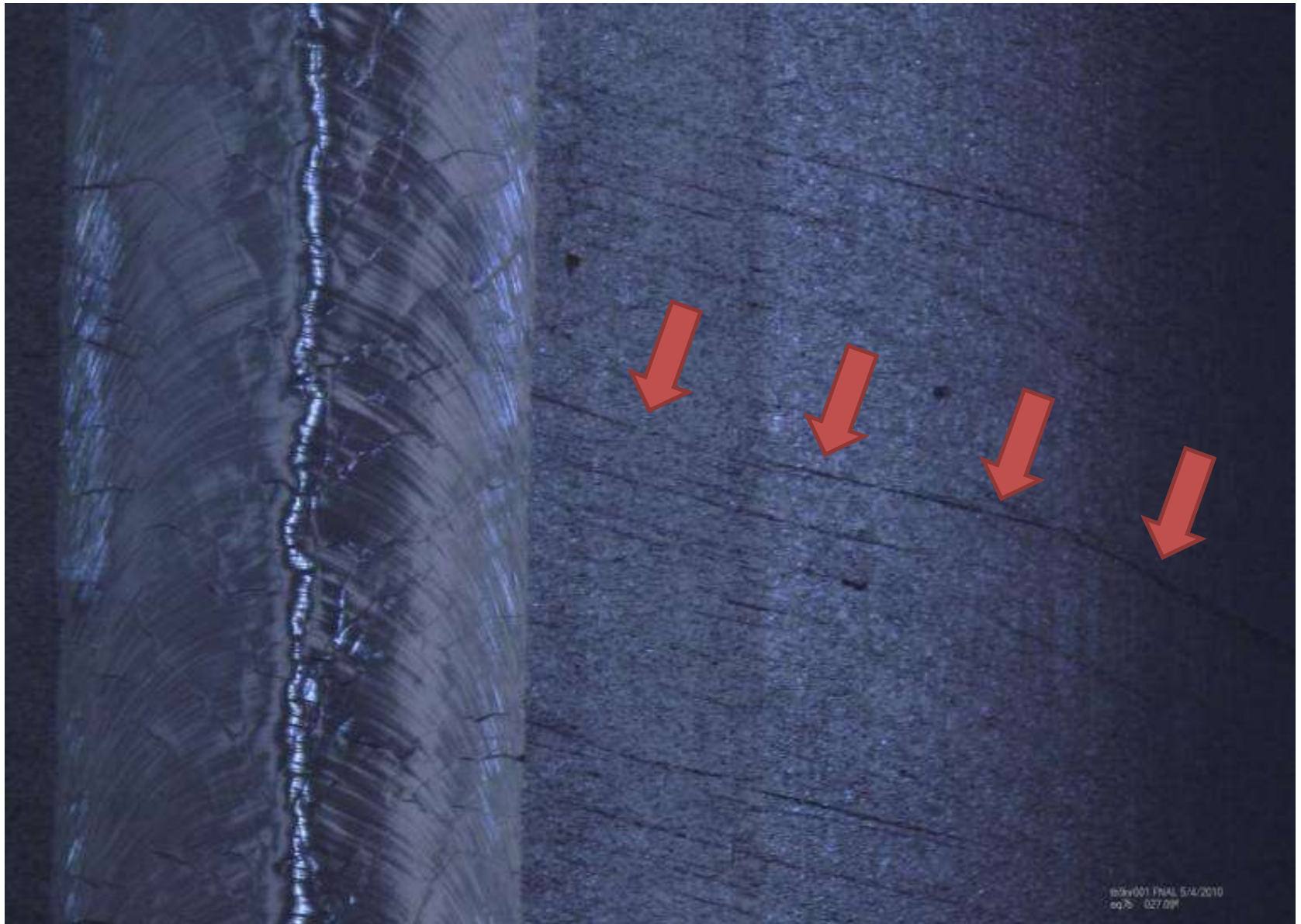
NR001: typical equator weld with non-typical horizontal lines. Not necessarily bad, could be related to the forming process and should be given some thought.
