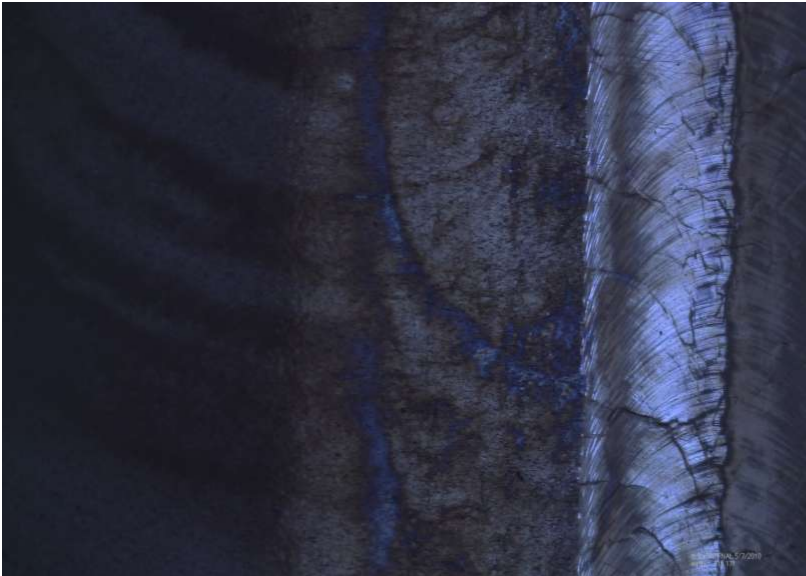
NR002: discolorations on equator weld, pictured is one of the worst extending ~20 deg and on both sides of weld. BAD – these discolorations should not be present
