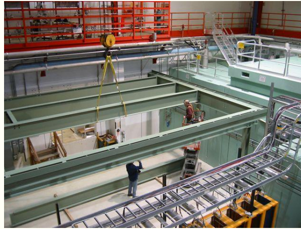
Erection of Laser Deck
