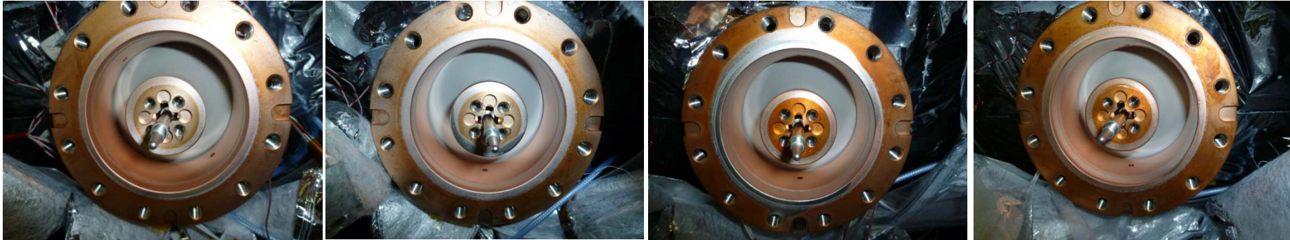
A1/MHI-05 (no leak)
