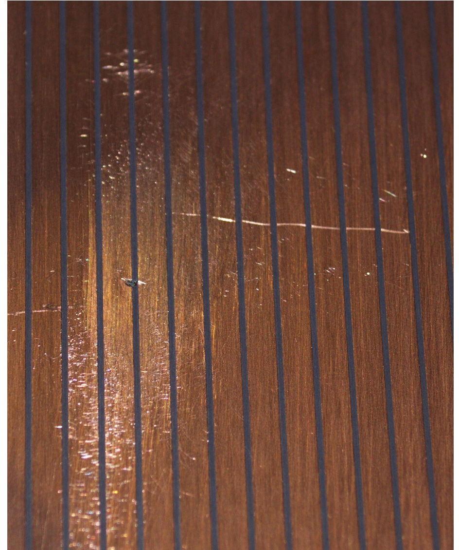
After grinding with very fine sandpaper
