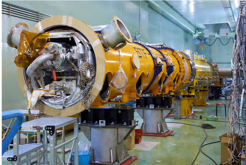
Figure 7-30: Placing Module-C and Module-A into the KEK-STF tunnel.
