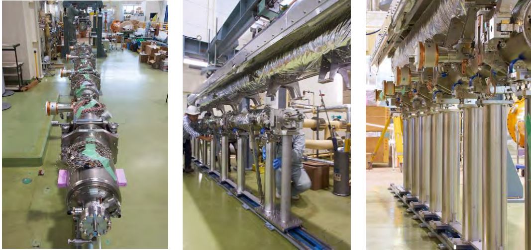
Figure 7-20: Placement of string cavities under the He-GRP.
