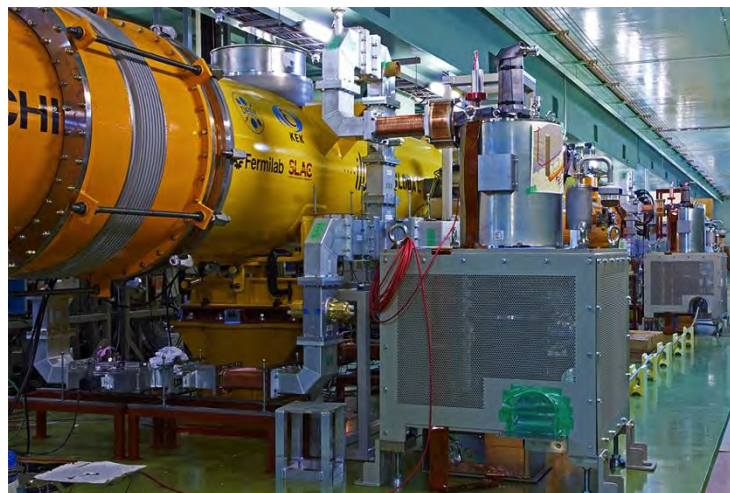
Figure 9-14: Picture of the DRFS in the tunnel.
