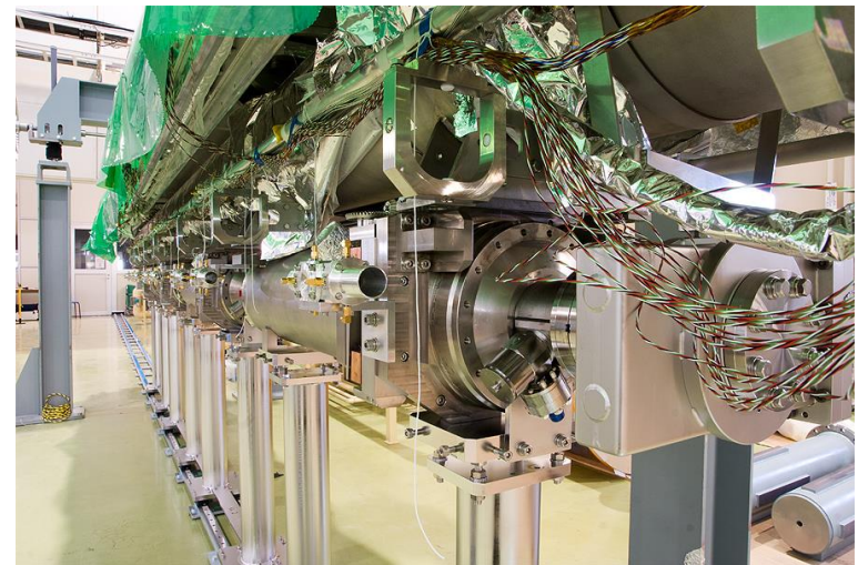
Cryomodule cold-mass assembly
