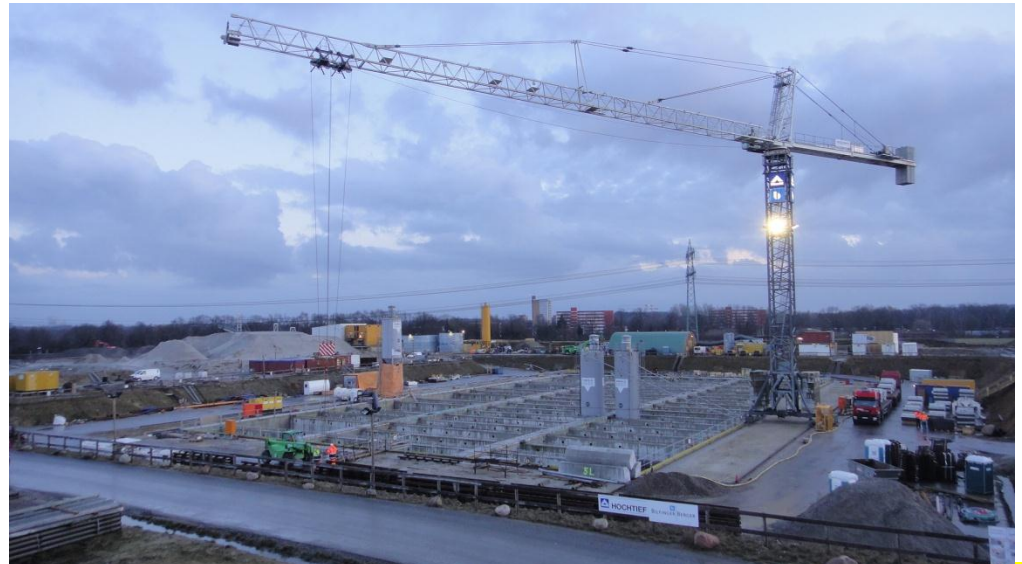
Construction of experimental halls is ongoing.
