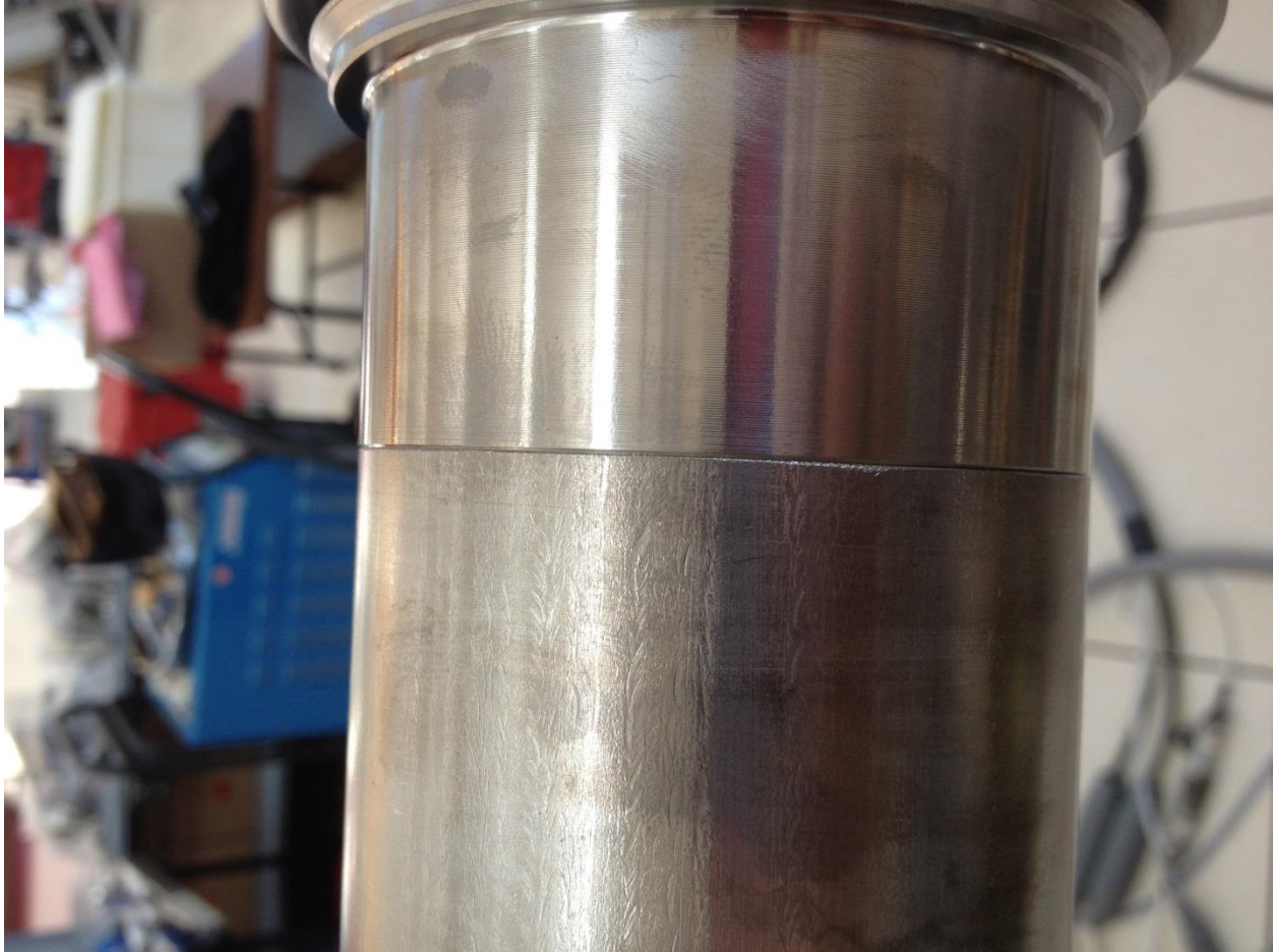
Figure 7: Two-phase line before welding
