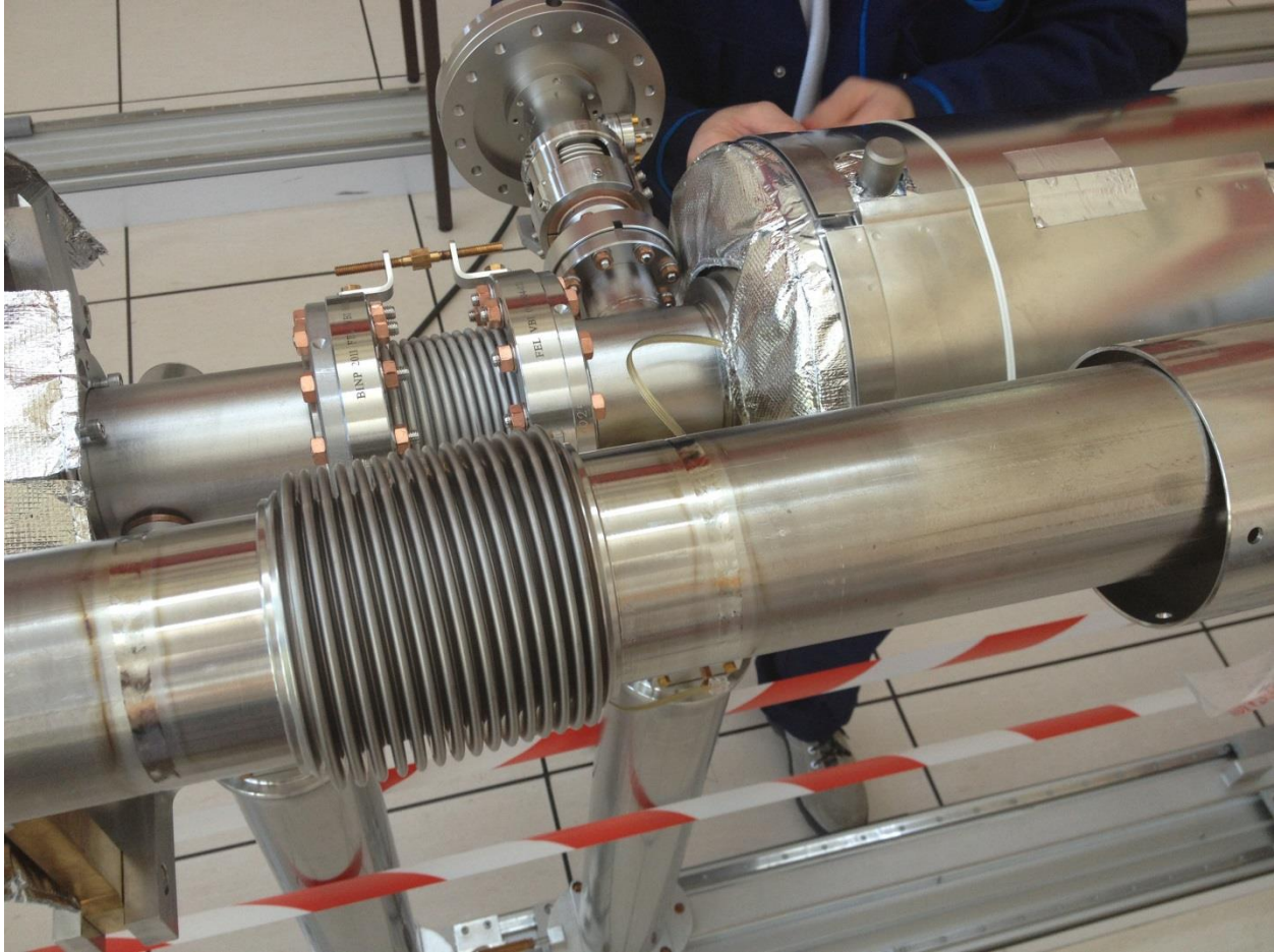
Figure 11: Completed welds and He vessel shielding.
