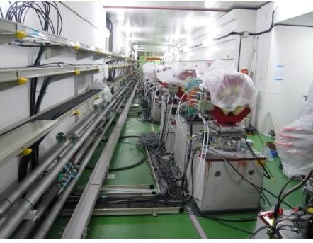
SLAC-built High Availability Power Supplies installed, connected and tested at ATF2
