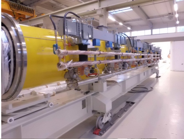
Waveguides with cooling tubes at module during installation test
