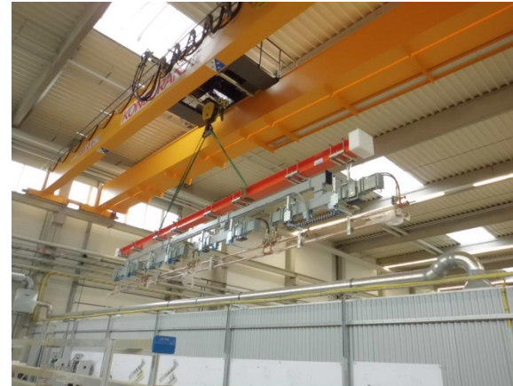
Waveguides at girder during installation test
