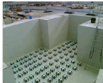
Example of usable PI (Biltz® B13W- vibration isolation rubber pad).
