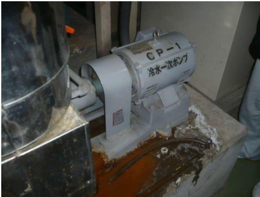
Water leak on the cooling pump for LINAC; repaired.
