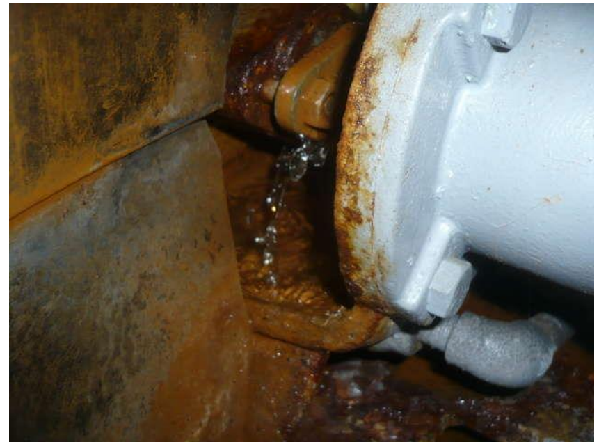
Water leak on the cooling pump for LINAC; repaired.
