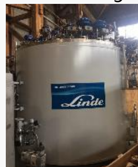
Helium recirculating tanks 2.5KW@4.5K cold box
