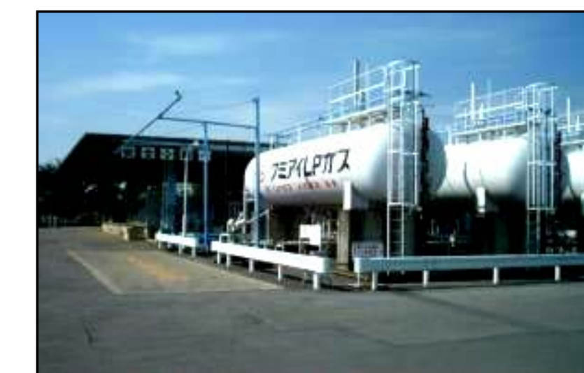
Photo 5: Horizontal cylindrical tanks
