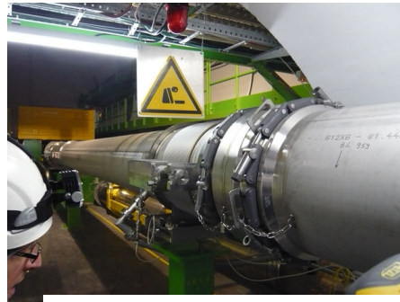
LHC beam dump window
