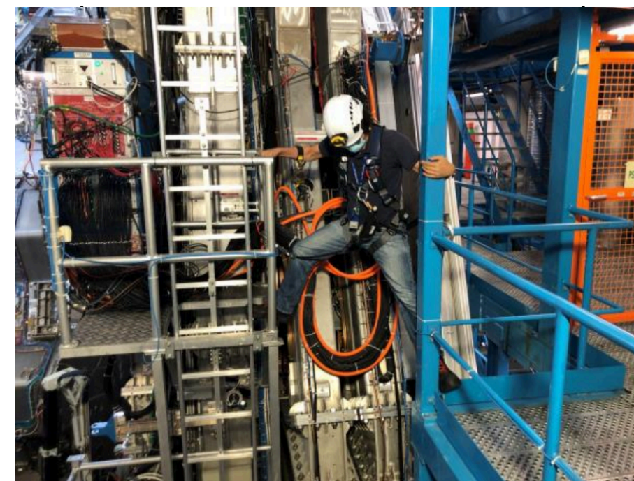
Me! jumping onto the detector at the 25m height to replace the electronics.
