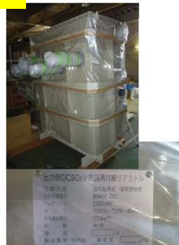
DC 90kV oscillator circuit for output
